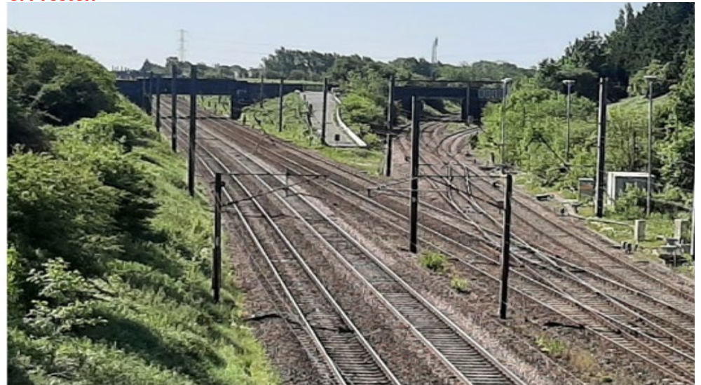
Existing rail line from Burscough (right) joining West Coast Mainline (left) south of Preston
